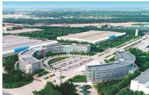
Weichai Power Technology Experimental Center Project
