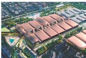
Beijing New International Exhibition Center Phase II Project
