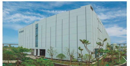
China Telecom Ningbo East Zhejiang Cloud Data Industrial Park
