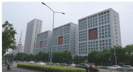
JD Cloud East China Data Center
