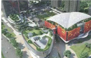
Zhuhai Hengqin Innovation Center Project
