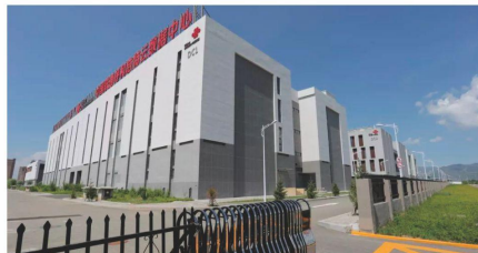
China Unicom Hohhot Cloud Data Center
