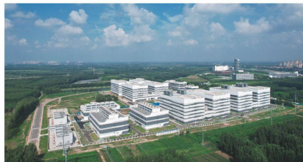
China Telecom Beijing-Tianjin-Hebei Big Data Center
