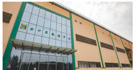
Hangzhou Iron and Steel Cloud Computing Data Center
