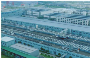
Yongsi Electronics (Ningbo) Chip Packaging and Testing Project
