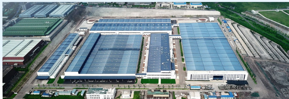
Intelligent Factory Photovoltaic Power Station
