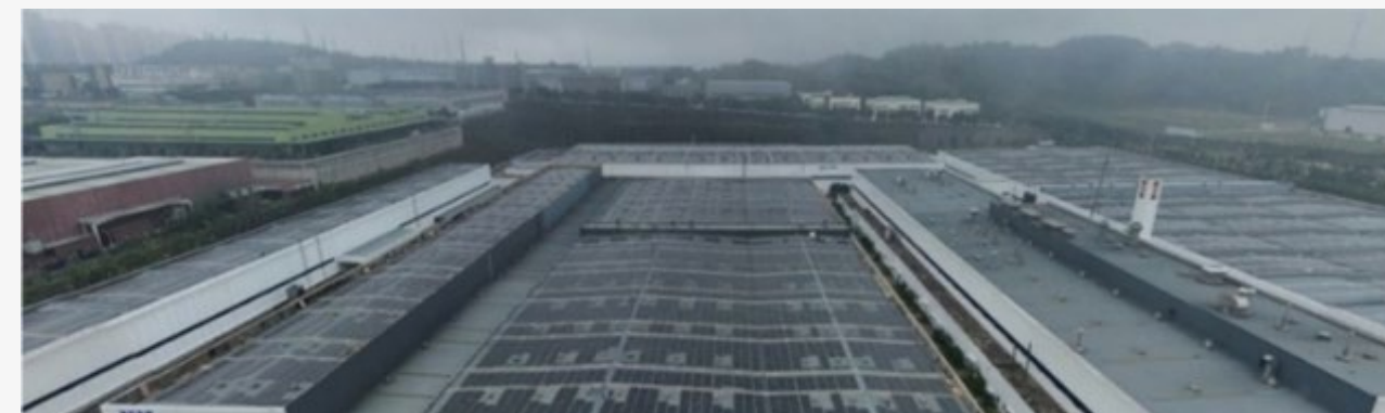
Solar photovoltaic power generation project
