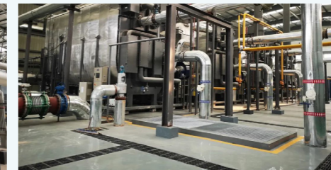
Supplementary-fired lithium bromide absorption heat exchange system
