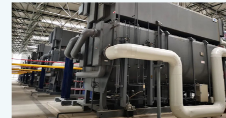
Supplementary-fired lithium bromide absorption heat exchange system
