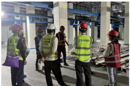
General Contractor Daily Safety Inspection
