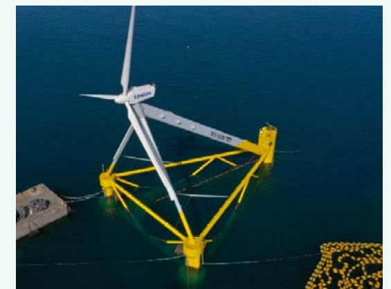
FWP dynamic cables for the X1 Wind project in Spain (an applied water depth of 90 meters)
