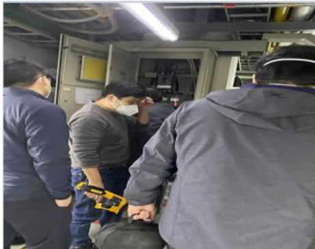
Site survey of Longhua G18-1F molding workshop
