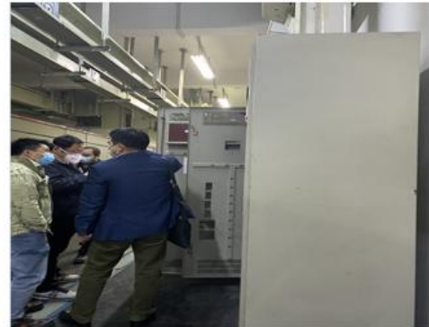
Site survey of Longhua E6-4F high voltage distribution room
