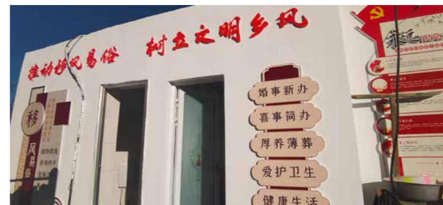
Chengdu Branch cooperates with Junyi Village in toilet renovation
