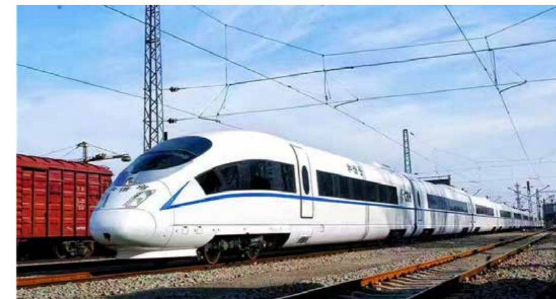
Intercity railway construction project in the Pearl River Delta
