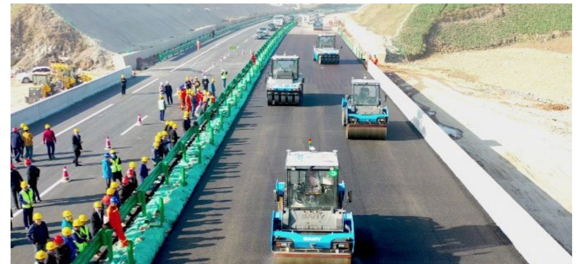
The unmanned fleet at a construction site
