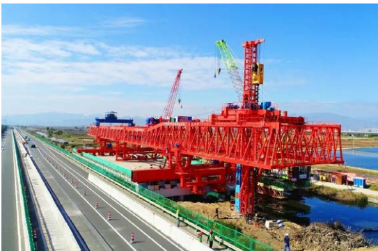
● 中铁工业研发的世界首台桩梁一体架桥机“共工号” “Gonggong No.,” the world’s first pile beam integrated bridge erecting machine developed by China Railway Hi-tech Industry Corporation Limited
