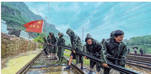
● 中铁七局紧急驰援太焦铁路抢险 China Railway No.7 Engineering Group Co., Ltd. rushed to restore Taijiao Railway
