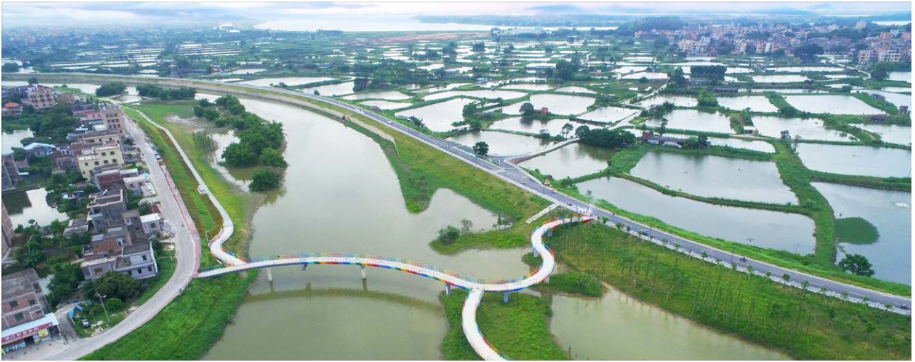
● 中铁上海局承建的鹤山市沙坪河综合整治工程 Comprehensive regulation project of shaping River in Heshan City undertaken by China Railway Shanghai Group Co., Ltd
