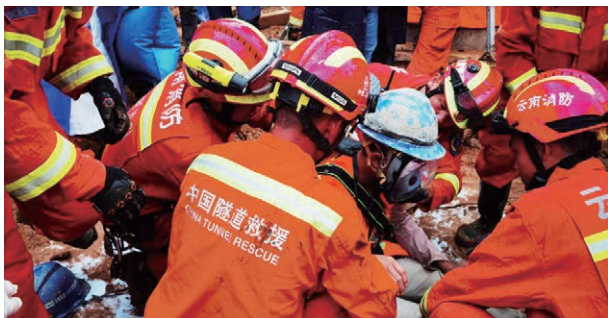
● 中国中铁救援队紧急驰援云南隧道坍塌抢险 CREC Rescue Team rushed to rescue people from the collapsed tunnel in Yunnan
