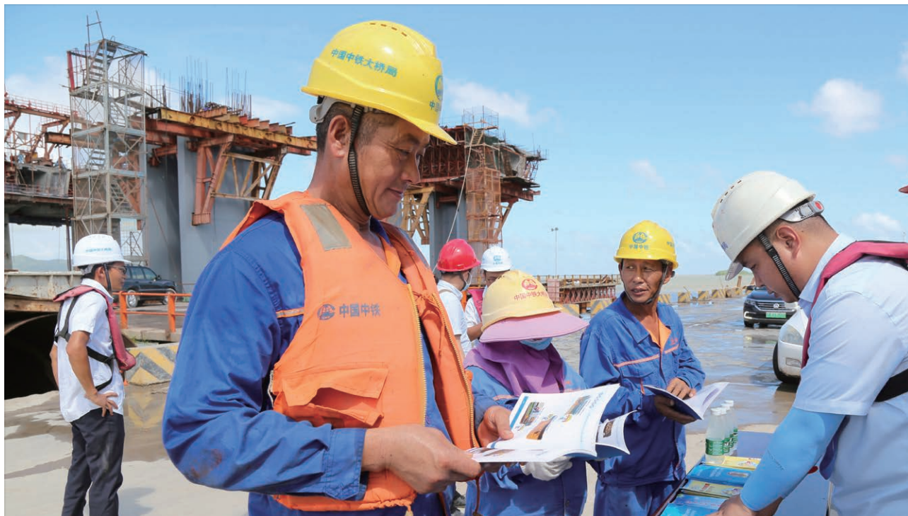
● 中铁大桥局珠机城际金海大桥项目部开展安全生产宣传教育活动 Zhuji Intercity Jinhai Bridge Project Department of China Railway Major Bridge Design Institute launched safety production publicity and education activities
