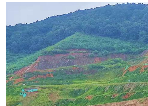
After slope greening
