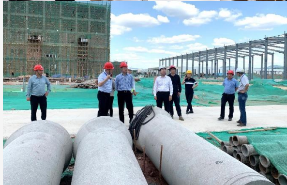
Special Inspections in 2021
