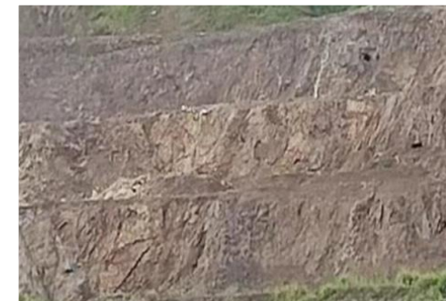
Before slope greening
