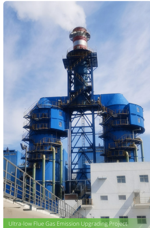
Ultra-low Flue Gas Emission Upgrading Project
