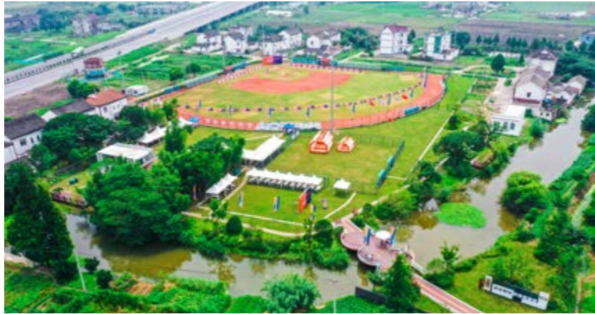
Hangzhou Branch helped build a beautiful countryside in Lindai Town, Pinghu
